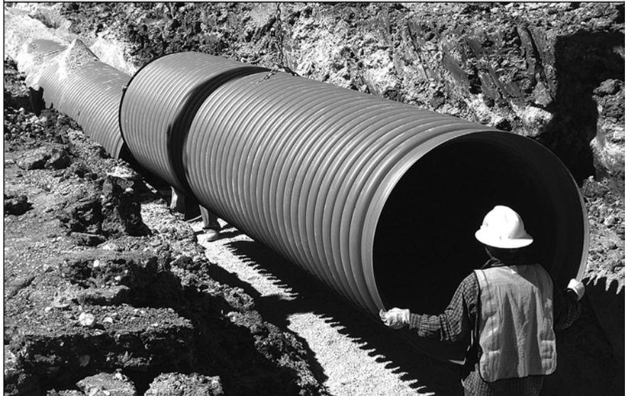
Available in dual wall and triple wall designs, HP Storm pipe exhibits superior strength and performance for storm sewer applications. Pennsylvania townships and municipalities can utilize the HP pipe under highways. HP Storm meets AASHTO M330 and ASTM F2736 and F2881.
